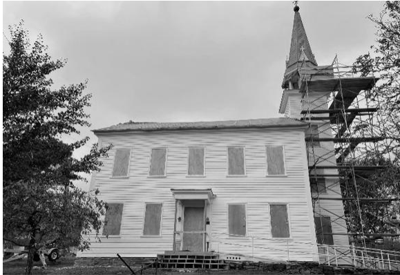
Renovation Underway - October 16, 2025
