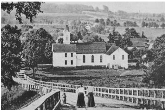
Methodist Episcopal Church Delanson, N.Y.
